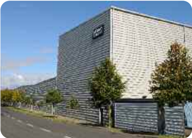
Instant UpRight Headquarters and Manufacturing Plant, Dublin, Ireland.
