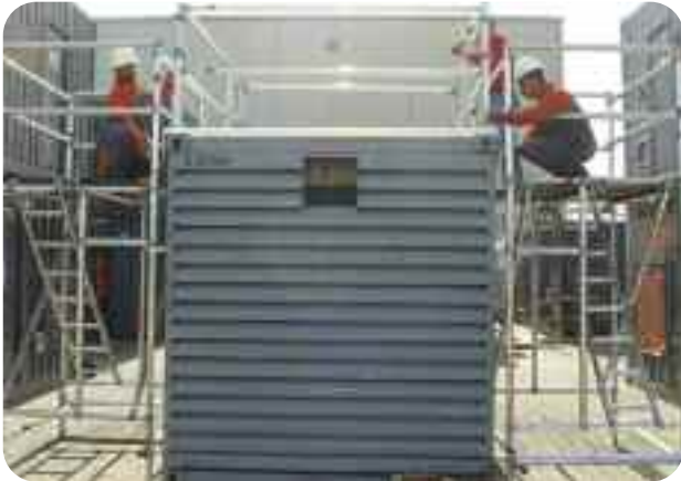
Edge Protection system for roofs. Supplied to Aggreko to fit 20ft containers housing generators in UAE and elsewhere across the globe.
