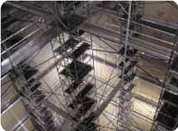
Partial view of the main tower structure at Manjung.
