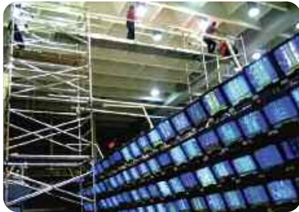
Roof access in TV studio.
