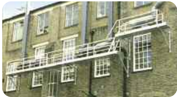
Split-level Spandeck Walkway provides Fire Safety Access on old building.
