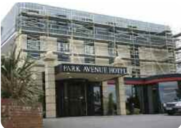
Aluminium Façade Scaffold - Park Avenue Hotel, Belfast.
