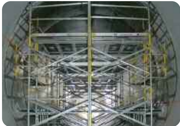
Standard tower components reconfigured for Wind Tunnel access.
