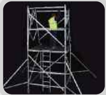
Once inside the boiler, each Snap-Out unit expands in seconds to provide a fully-braced 2m cubic tower module. Ladders and platforms are quickly fitted before adding the next Snap-Out module.
