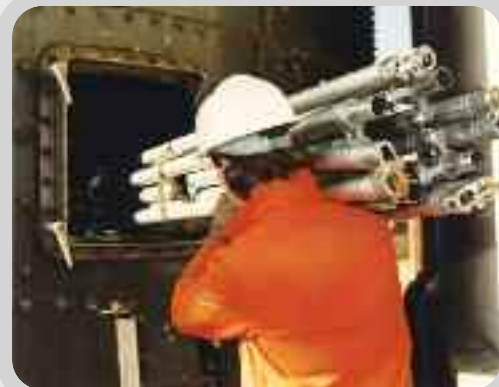
Folded one-piece Snap-Out units pass through a small manhole and expand into rigid and fully-braced 2m cubic tower modules in seconds!
