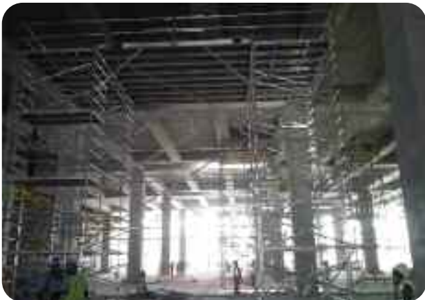
7.2m x 5m x 5m rolling stage in Abu Dhabi Midfield Terminal Airport.
